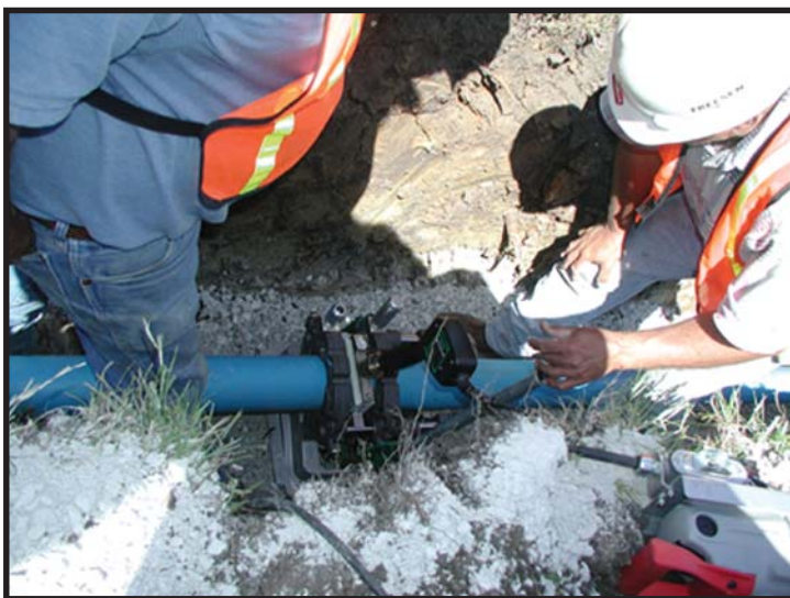
Delaware County RWD #10-Pictured to the left is a close up of workers fusing a water line.
