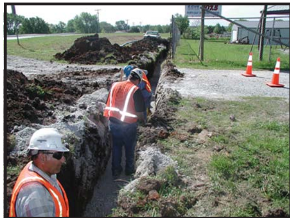
Delaware County RWD #10- Workers are laying a new water line.
