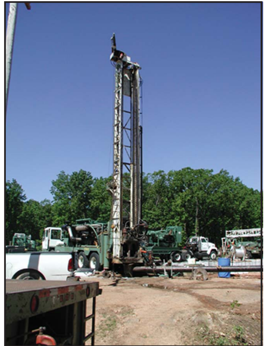
Delaware County RWD #10- Drilling Well #2
