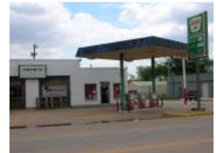
Review of local communities' wellhead protection plans helps assess potential sources of contamination.
