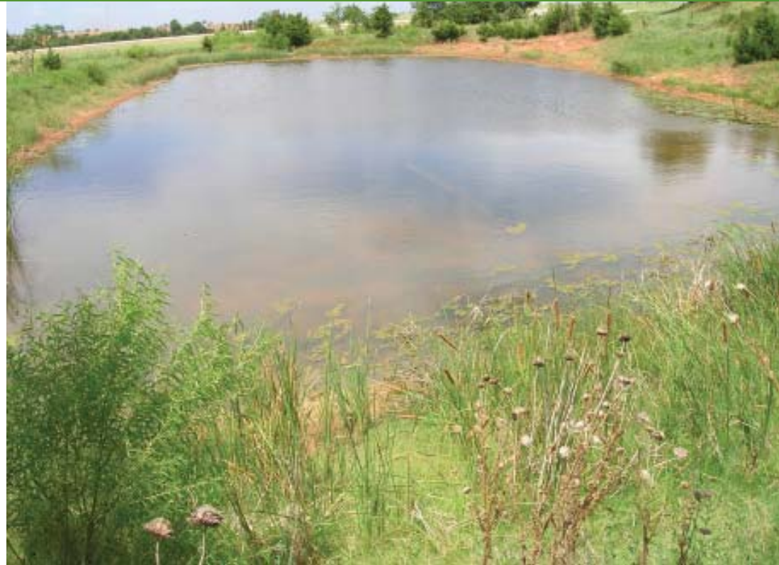
A total-retention lagoon that is not well maintained.
