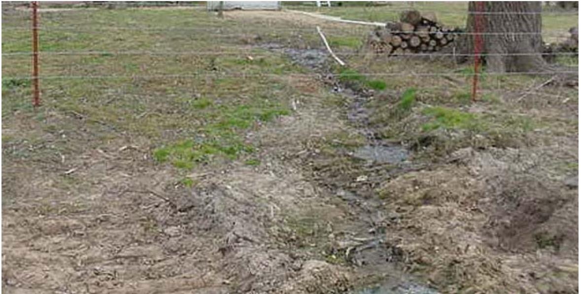
*Sewage surfacing from a failing septic system.*
