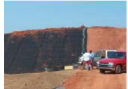
Pictured here is a slide slope of a lined cell under construction.
