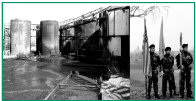
Parawax Before Remediation
