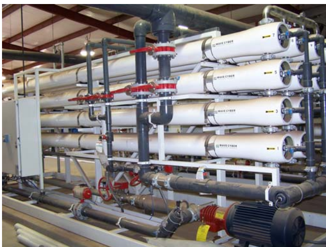
Figure 4 – Cherokee reverse osmosis system
