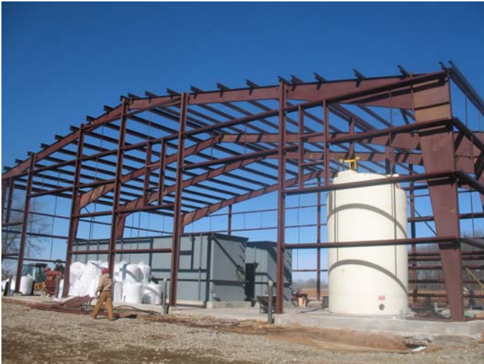
Figure 6 – Actiflo plant construction.
